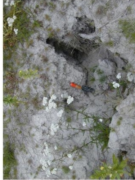
Picture 2. Deep erosion hole on the untreated part of the slope
