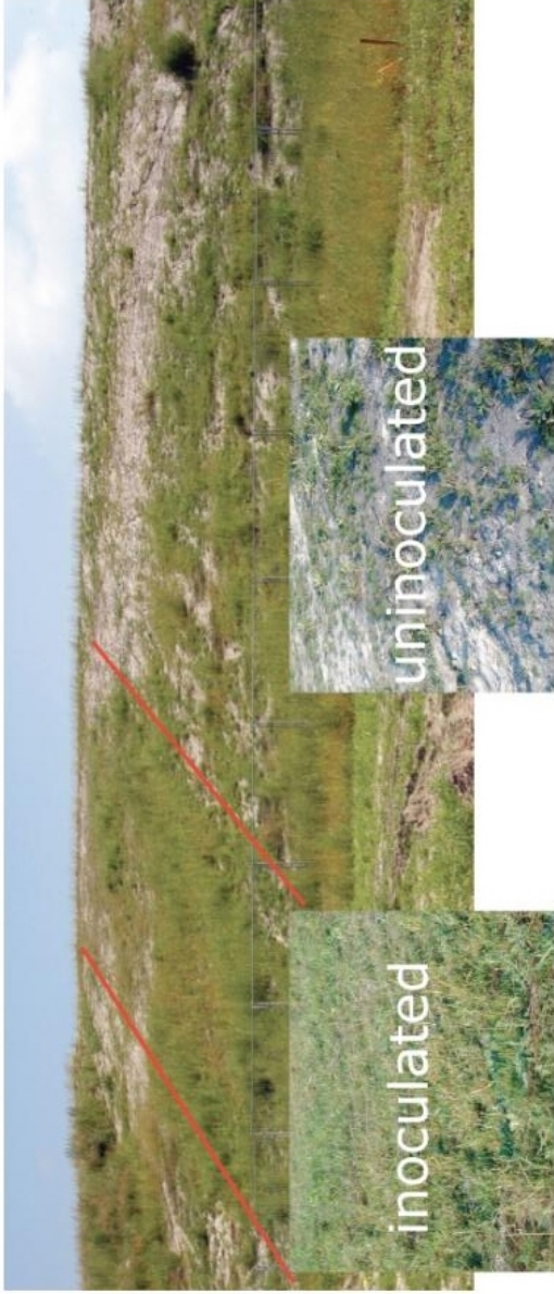
Picture 1. Noise barrier near Breda. The stroke between the two red lines was treated with mycorrhiza at sowing
